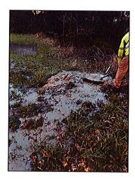
The staff was able to quickly respond with a jet truck and equipment through the cleared easement. Once the clog was removed the area needed to be cleaned up and stabilized. It was determined that large amounts of grease were to blame for the blockage.
