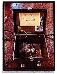
To better control the oxygen distribution throughout the aeration tanks we are planning to upgrade our dissolved oxygen probes and programming. Our maintenance team was able to build the power supply electrical boxes in house. The programming of the instrumentation will be done through an outside vendor.
