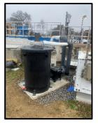
The Pure Air Carbon odor control system has been installed on the gravity thickeners and has been placed into service. The units have been on-line for less than a week and have been effectively eliminating the odor from the tanks.
