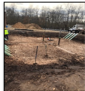
The spent media being removed from the biofilter.
