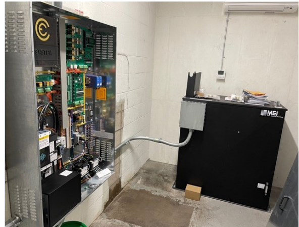
Town Hall Elevator Control Box and Hydraulic Pump
