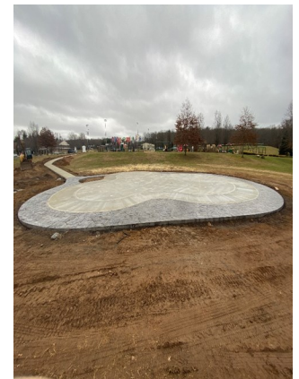
We Just finished Side walk and Stamped concrete around the Spalsh Pad
