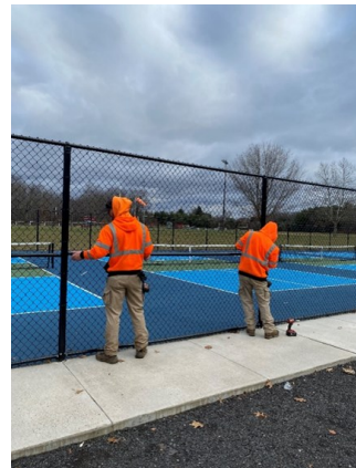
Added a center rail to pickleball for fence strength.
