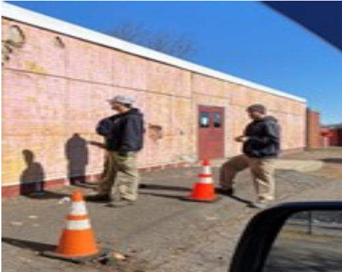
Parks Crew removed old rotten T-111 walls from the Old Orchard Hill School portables and replaced it
