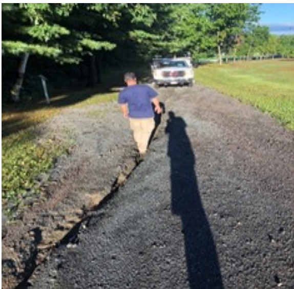
We spend Aprox $3,000 a year in material alone to maintain stone dust trails in SW because of heavy rains that cause wash outs. After a heavy rain it takes two mainatiners all day to repair them
