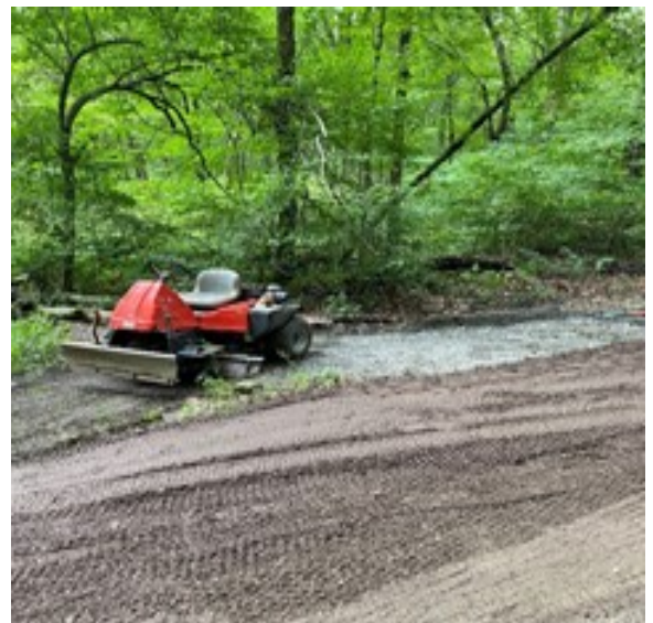
We spend Aprox $3,000 a year in material alone to maintain stone dust trails in SW because of heavy rains that cause wash outs. After a heavy rain it takes two mainatiners all day to repair them
