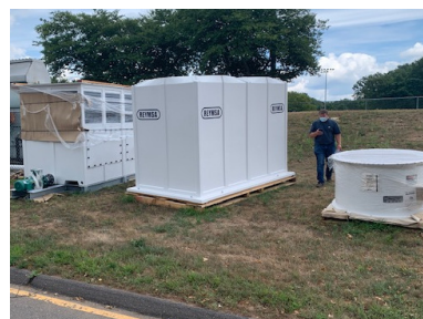
Cooling Tower Assembly at the Community Center
