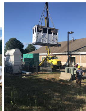
Cooling Tower Assembly at the Community Center
