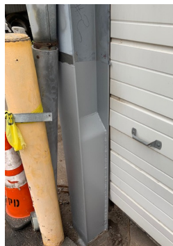
I-Beam Repairs at the Town Garage
