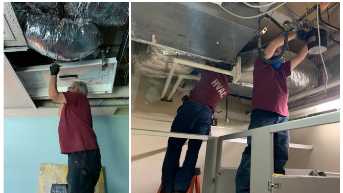
Community Center Heat Pump Replacements
