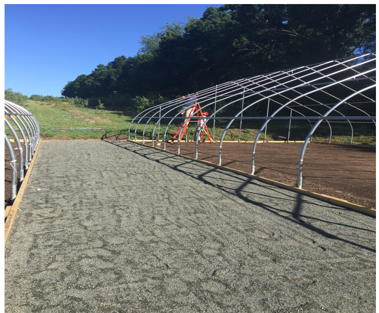
High Tunnel construction at the Avery Gardens site – sonotubes placement for concrete footings above and frame erection below
