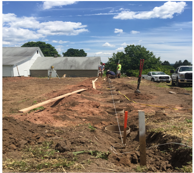
High Tunnel construction at the Avery Gardens site – sonotubes placement for concrete footings above and frame erection below
