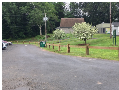
Installed heavy-duty wooden guard rails at the indoor batting building to better delineate parking from lawn areas at parking lot and provide a more secure safety barrier/separation of vehicular and pedestrian traffic and prevent unauthorized parking. Also replaced the post and rail fence with the same guard rail system at VMP.
