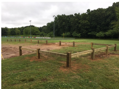
Installed heavy-duty wooden guard rails at the indoor batting building to better delineate parking from lawn areas at parking lot and provide a more secure safety barrier/separation of vehicular and pedestrian traffic and prevent unauthorized parking. Also replaced the post and rail fence with the same guard rail system at VMP.
