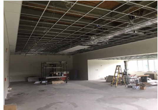
Wapping cafeteria remodeling – new walls are up, rough electrical, A/C and ceiling grid complete.
