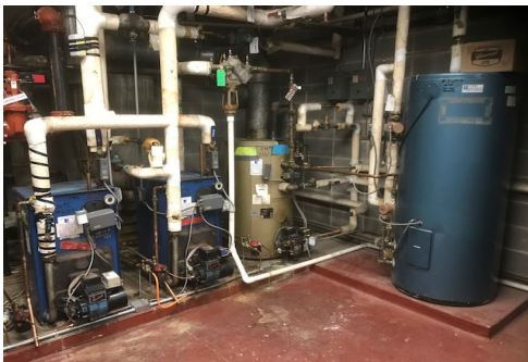
Old Boiler and Storage Tank at the Police Department
