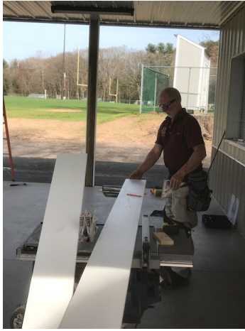
Mike Costa at Rye Street Concession Stand Fabricating PVC Trim to Wrap Exposed Wood Roof Support Columns
