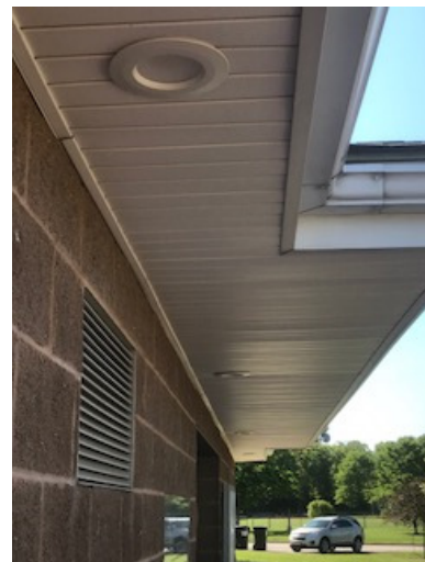
LED Soffit Fixtures at the Press Box
