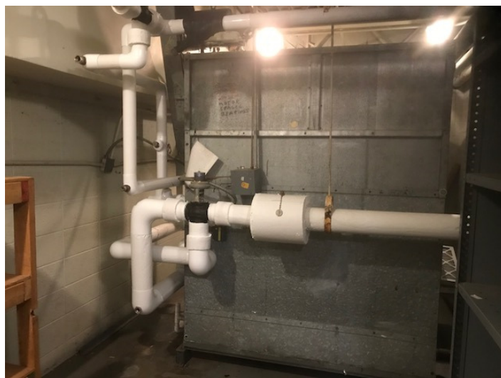
Newly Insulated Cold Water Piping on Air Handling Unit at Town Hall
