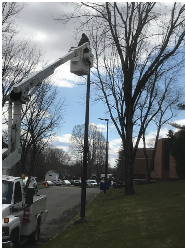
Electrical Contractors Inc. installing new LED Parking Lot Lights at the Library
