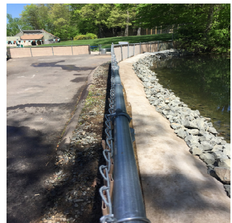
Installation of concrete cloth erosion control at the back pond at VMP
