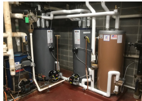
New Hot Water Boiler, Piping, and Storage Tank at the Police Department
