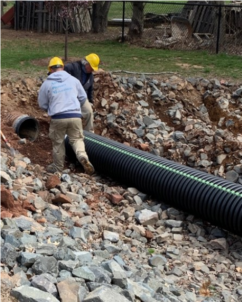
Parks Crew eliminated a large swale behind Eli Terry School to make a safer area behind the school. They added 120 of 18" ADS pipe, and 276 yards of material. They also regraded and seeded that space.
