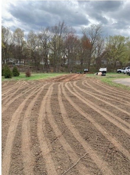
Parks Crew eliminated a large swale behind Eli Terry School to make a safer area behind the school. They added 120 of 18" ADS pipe, and 276 yards of material. They also regraded and seeded that space.
