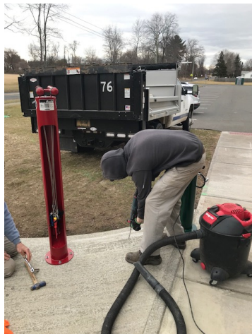
Parks crew installs the SWW&WW bike repair station on new concrete pad at the new restroom facility at Nevers Park
