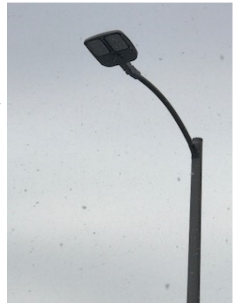
Right: New LED Style Parking Lot light Pole Fixture using 86 Watts
