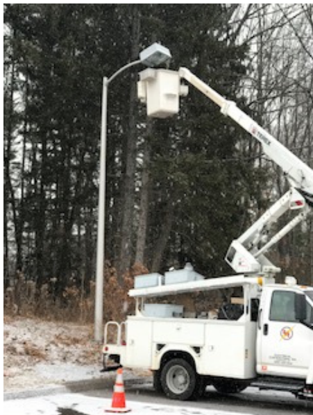
Left: Original Induction Style Parking lot light pole fixture using 225 Watts at Town Hall
