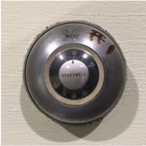
Left: Manual style pneumatic thermostats removed in Meeting, I.T. and Lunch Room at Town Hall
