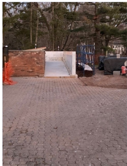
Concrete Ramp Poured
