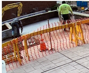
Patio Concrete Section Poured
