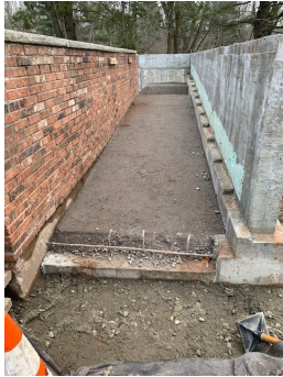
Ramp Walls Erected
