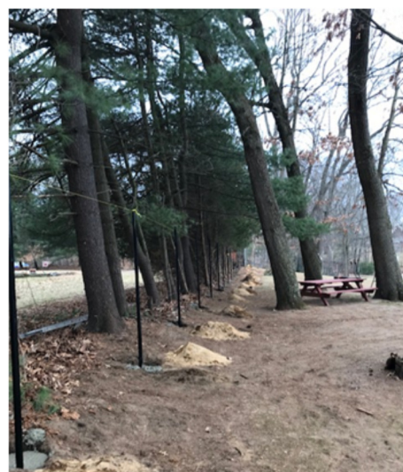
Parks crew takes advantage of the recent mild winter conditions to install a new privacy fence along the private property line of a close abutting neighbor to Veterans Memorial Park. The old wood stockade fence had rotted and is being replaced with a 6 foot high chain link fence with privacy slats.
