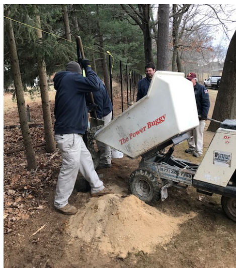
Parks crew takes advantage of the recent mild winter conditions to install a new privacy fence along the private property line of a close abutting neighbor to Veterans Memorial Park. The old wood stockade fence had rotted and is being replaced with a 6 foot high chain link fence with privacy slats.
