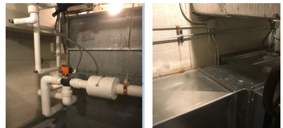
New DDC Valves and Ductwork to Precisely Control Heating and Cooling in Council Chambers
