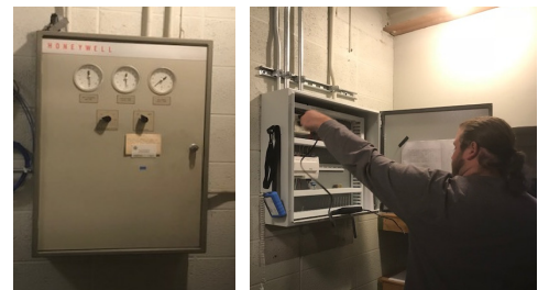
Old HVAC Pneumatic Controls Being Replaced by New Direct Digital HVAC Controls for Council Chambers
