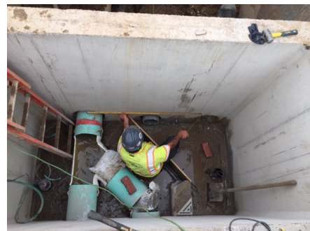
Photo: Sullivan Avenue Siphon inlet structure being built.
