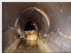
Photo: These images were taken by the WPC staff using a CCTV inspection camera on Griffin Rd. The sewer pipe is failing and beginning to collapse.
