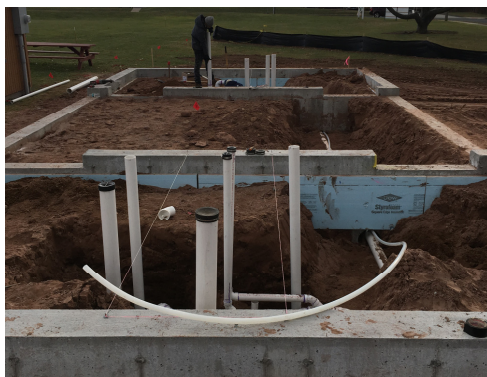
Nevers Restroom project— rough plumbing installation
