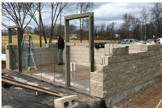
Nevers Restroom project— block wall construction 1
