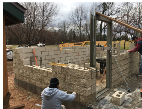
Nevers Restroom project— block wall construction 2
