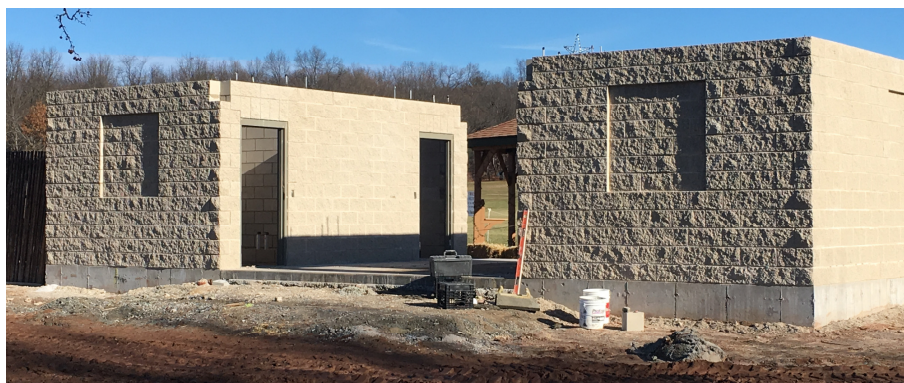
Nevers Restroom project – block wall construction completed
