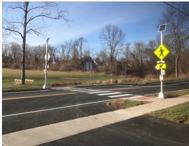
New solar-powered crosswalk signals at Nevers Park
