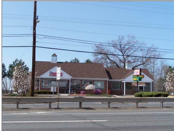
With overhead wires:
