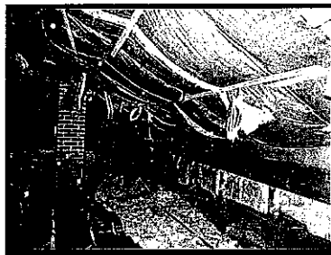
lower attic- insulation covering rafters
