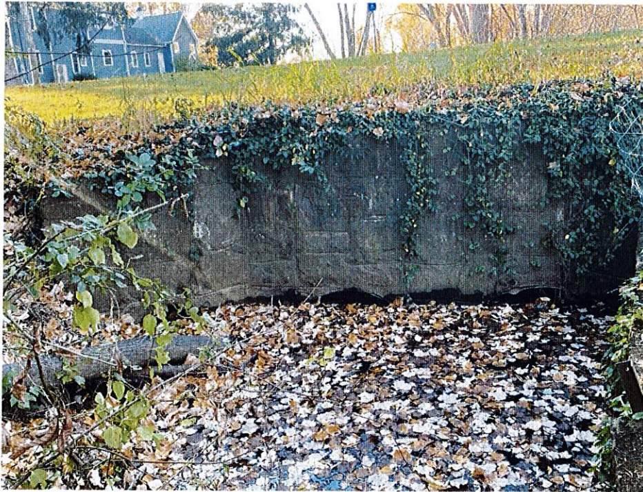
Figure 7: Newberry Brook culvert under Main St looking south, 11/8/2021. The tops of the two drainage pipes are just visible above the water level on the upstream side.
