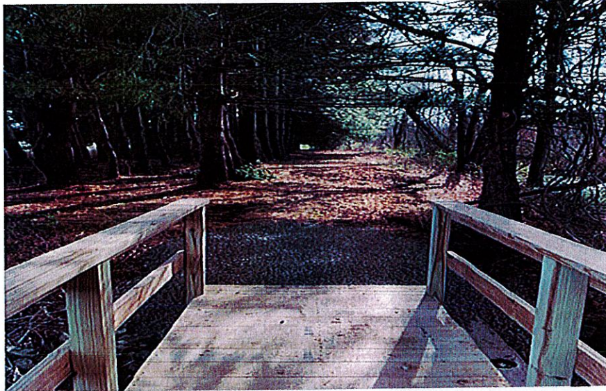
The new bridge at the South Windsor Fishing Derby pond off Frazier Fir offered access to the entire pond for participants of the Fishing Derby
