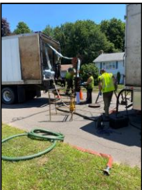
Image shows crews inserting the new sewer lining on LeFoll Blvd.
