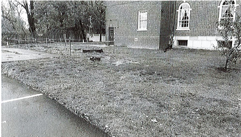
South side of Library; green door is ADA entrance
