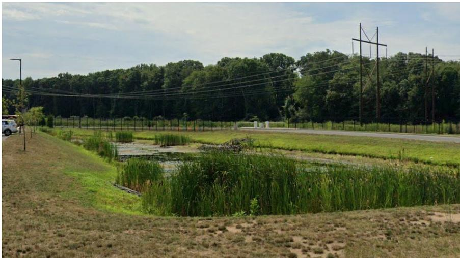
*Detention ponds are a stormwater management strategy that seeks to collect and infiltrate stormwater on-site.*
