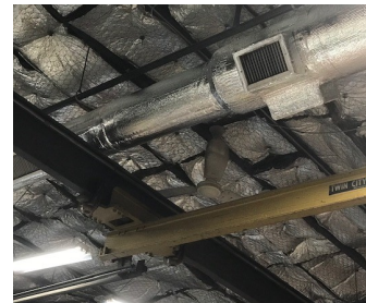
Insulated Ductwork in Mechanic Bays at the Public Works Garage
