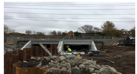
Buckland Road Culverts for Plum Gulley Brook
