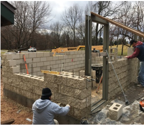
Nevers Restroom project – block wall construction
