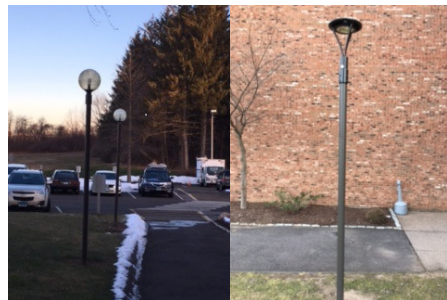
Left: Old Fluorescent Fixtures Right: New LED Fixtures
