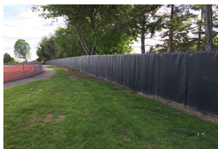
Sound & visual barrier fence installation to buffer abutting neighbors from High School stadium
