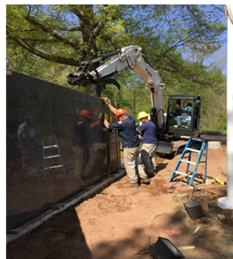
Granite panel installation at Memorial Wall @ VMP
