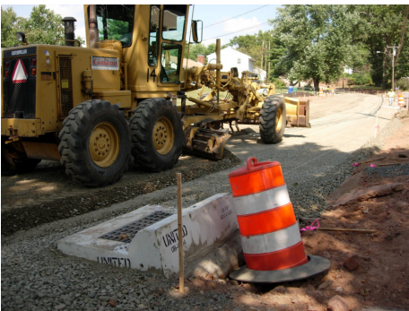
Grading new road base on Dart Hill Road at the sharp bend at the bottom of the hill
