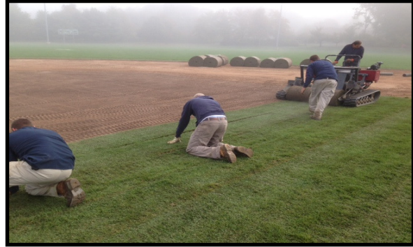
Rotary Baseball Infield Renovation – sod installation
