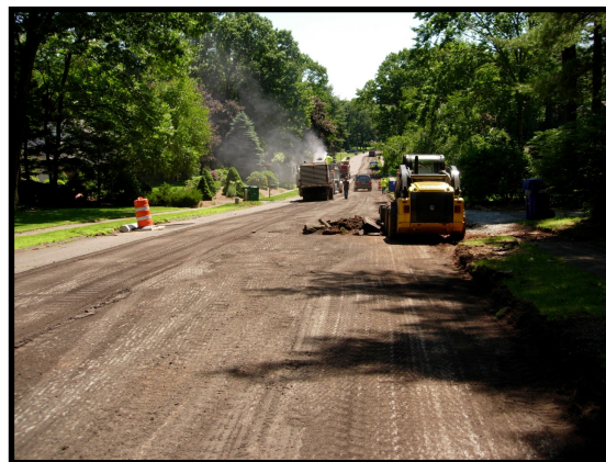
Milling old pavement on Berle Rd
