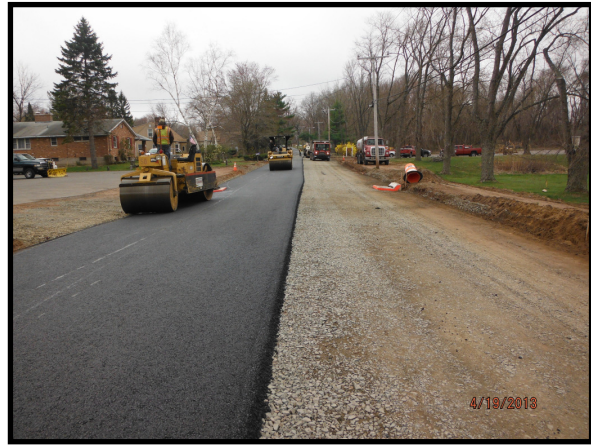
Long Hill Road – Stone base and first course of asphalt pavement
