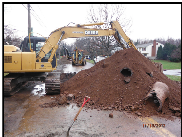
Foster Street Extension – Removing old pipes and installing new drainage pipes
