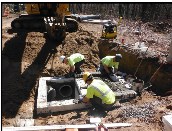
Strong Road - constructing a new drainage catch basin
