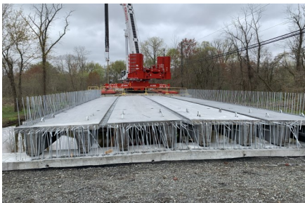
Main Street Bridge – New Beams Being Set
