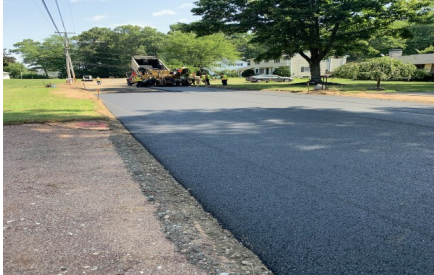
Ident Road was reconstructed with new drainage, base and pavement.
