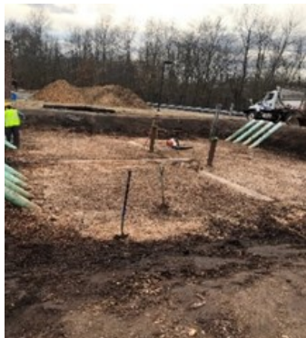
The spent media being removed from the biofilter
