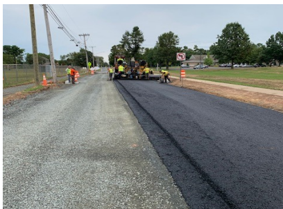
New base and pavement on the south section of Nevers Road
