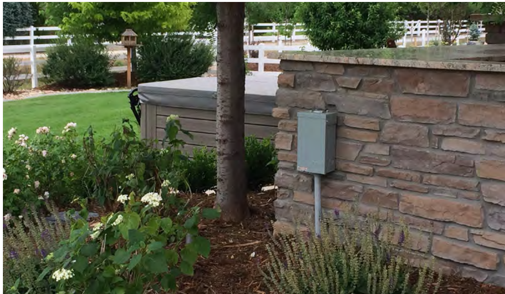
Figure 10-1-2: Though within 50 feet, this disconnect cannot be seen from the hot tub location.
