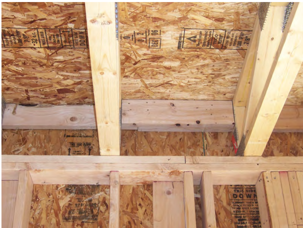
Figure 4-3-4: Floor trusses don't have a band joist, so the connection methods from the IRC do not apply. Alternate connections are provided by the Structural Building Components Association at its website, sbcindustry.com .
