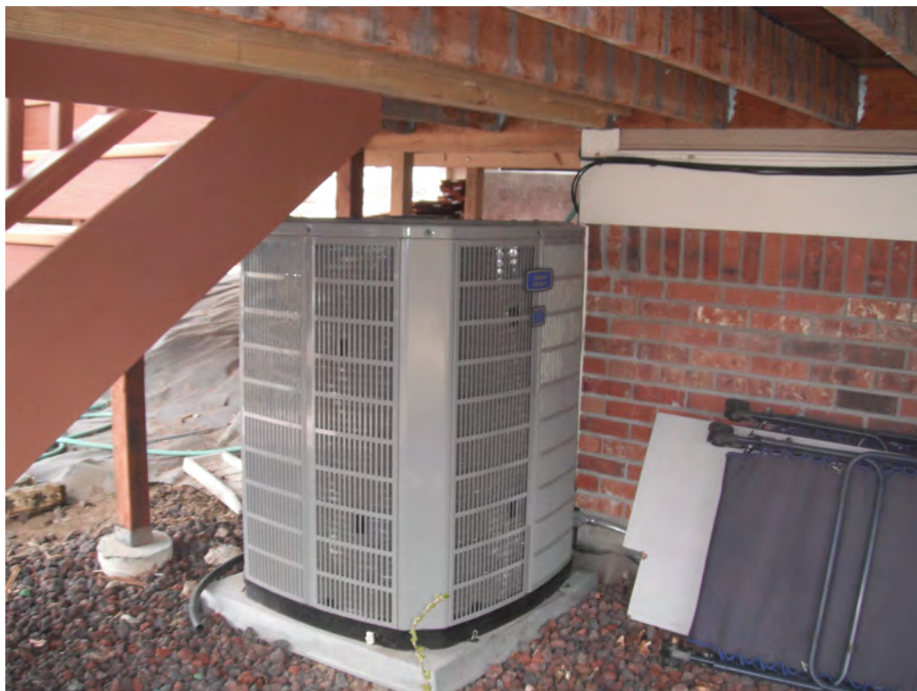
Figure 2-4-2: It could be interpreted that an air conditioning compressor must have a 6.5-foot-high clearance around it, but that could also be considered unnecessary. Manufacturer’s installation instructions, however, will require a clearance above the unit for airflow, usually between 12 and 48 inches depending on the size of the unit.
