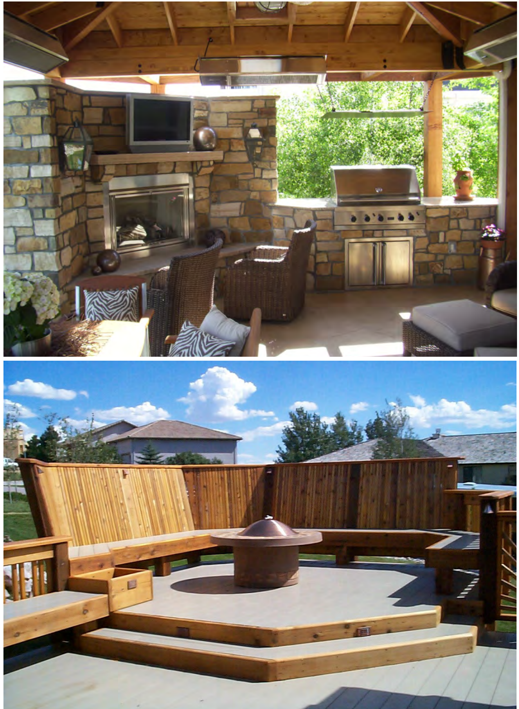
Figures 9-1-2 and 9-1-3: A guard isn't always a guardrail, and sometimes doesn't even resemble a guard. A built-in BBQ kitchen, a planter box, a half wall, a fireplace, a bench, and a privacy wall are all examples of features that can serve other functions but still act as a barrier to a fall. These features would need to meet the loading, minimum height and opening restrictions required for guards, when functioning as a required guard.
