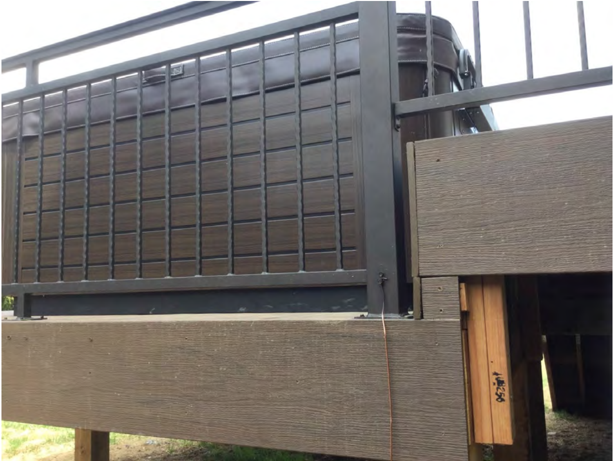
Figure 10-1-4: Hazards related to occupant contact, such as safety glazing, switches, disconnects, lighting, and metal objects, follow a 5-foot reach rule. The clearances described in these sections are very similar to those required for luminaires, previously discussed. Bonding metal guards, as shown in this photo, is not usually done by design, as it is aesthetically displeasing and easily removed by unaware occupants after the inspection passes. When designing a hot tub installation, it is recommended to simply design a clear 5-foot horizontal space around the tub free from all the aforementioned items.
