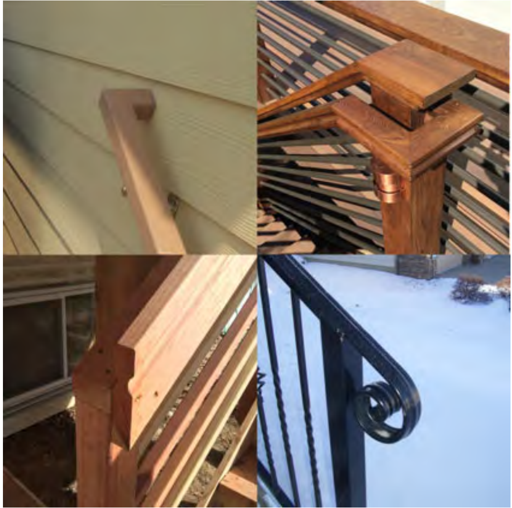
Figure 9-2-3: To avoid catching purse straps, loose clothing or articles held by the user, handrails must terminate into a post or wall or be otherwise returned to face an alternate direction.
