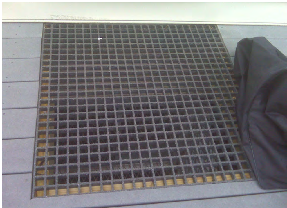
Figure 2-6-3: A drop-in panel, such as this composite material, is lightweight enough to remove with a simple push, yet strong enough to resist live loads. This is all that must be satisfied, regardless of the design.
