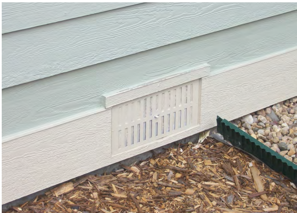
Figure 2-3-8: Though this one is nearly painted shut already, it's also right where a ledger would connect. Ledgers must be severed at vent locations and joists laid out on either side. Shallower blocking spaced away from the wall can be installed between joists to support angled decking if necessary.
