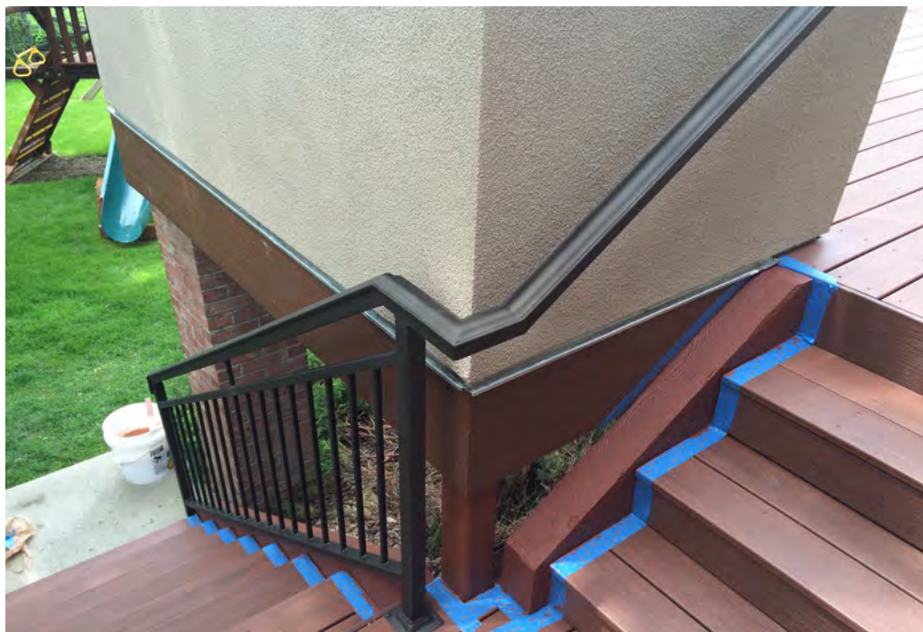
Figure 9-1-1: Though the handrail shown is not required to be continuous around the corner, this installation provides a good example of how a handrail can be both stand-alone and incorporated into a guard. The guard can be typical railings or the wall adjacent to the upper stairs. In all cases, they perform their respective duty.
