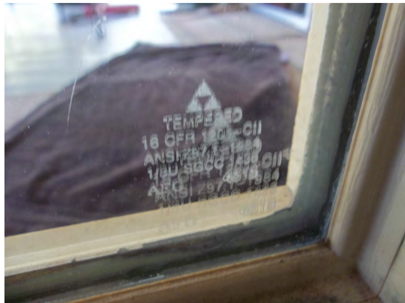
Figure 2-5-1: For tempered glass, a permanent etching is typically provided on the glass that lists the necessary information. They are as hard to read in person as they are in this photo.
