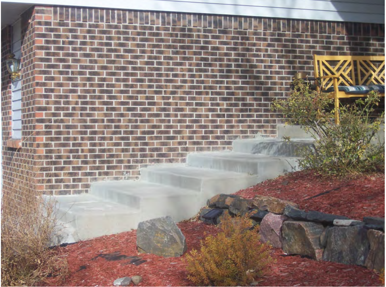
Figure 9-2-2: Though a similar entry to the other example, this flight of stairs requires a handrail. The treads are deep horizontally but not enough to be landings.
