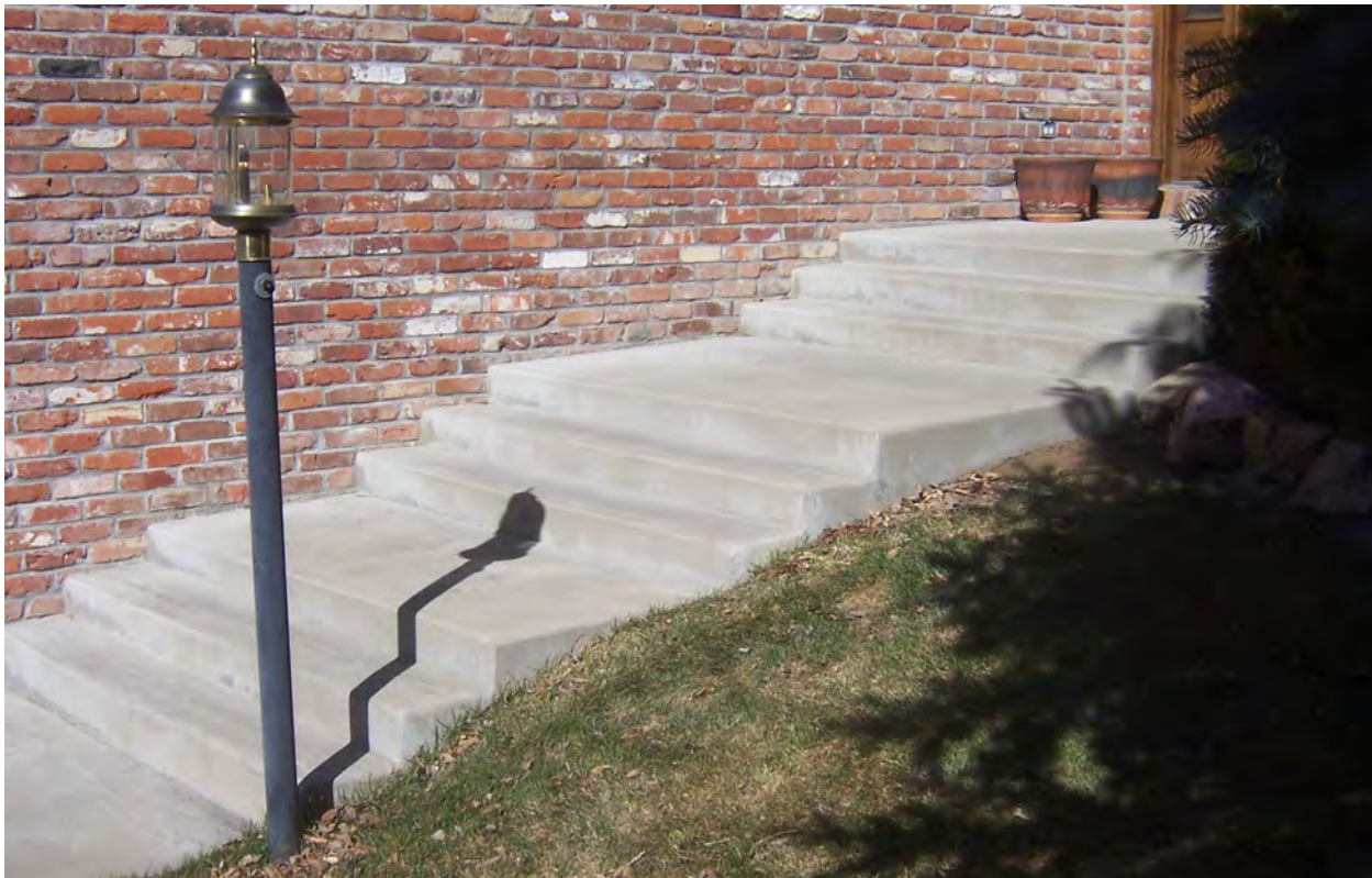
Figure 9-2-1: Where a handrail may not be desired, possibly for architectural reasons, a series of three rise stairs with intermediate landings can be used. With less movement between resting places on the landing, a handrail can be omitted.
