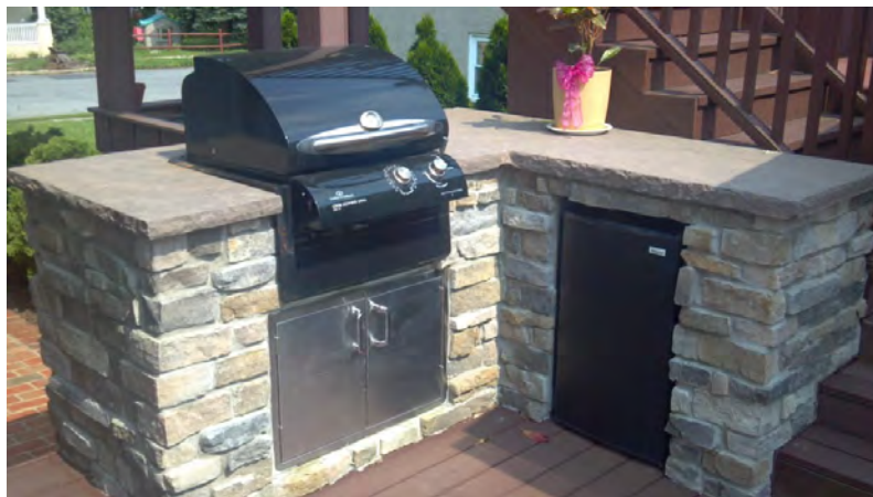
Figure 10-2-1: If on the right-side countertop, this grill would likely have been too close to the guards.
