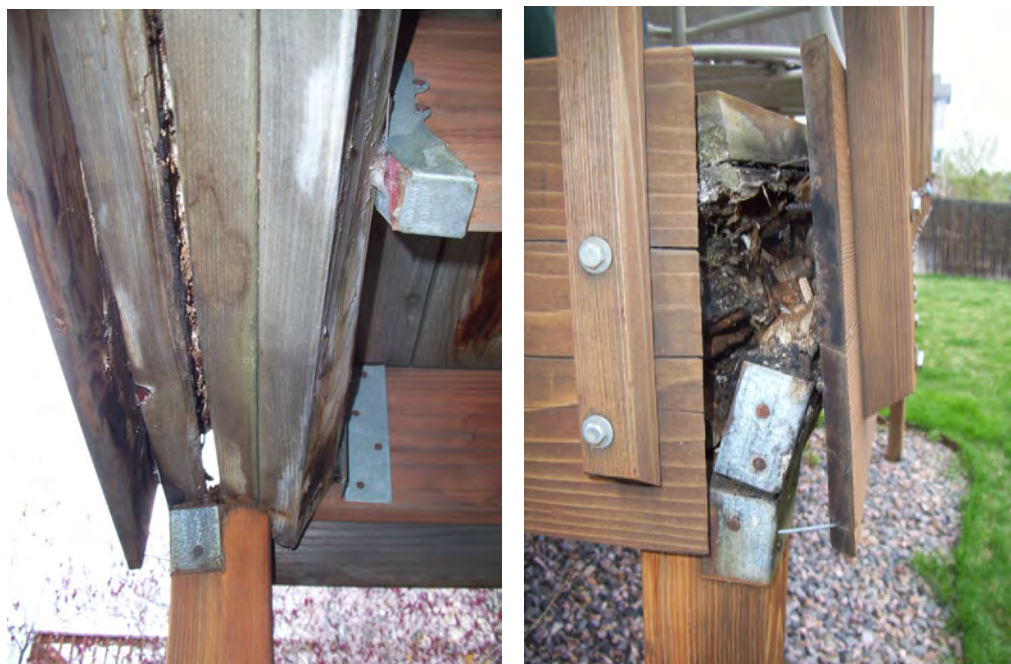
Figures 3-1-1 and 3-1-2: Though this deck is 5 feet above grade, the 3-ply, wood, non-treated beam is able to trap water between the plies. This inhibited drying and resulted in structurally catastrophic decay.
