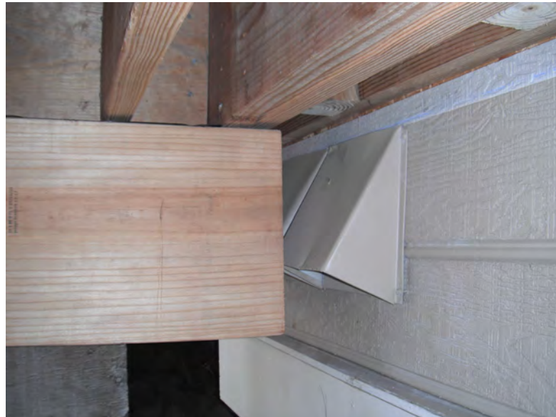
Figure 2-3-3: Similar to IRC Figure G2407.6.1(1), above, combustion air can come from under a deck. However, the airflow to the openings can't be obstructed. The beam shown here does not obstruct airflow. The overall deck design must be considered to determine if sufficient airflow can move under the deck.
