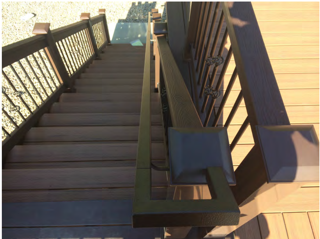
Figure 8-1-5: This 19-rise single stair flight is at the limit of vertical height before a landing is required.
