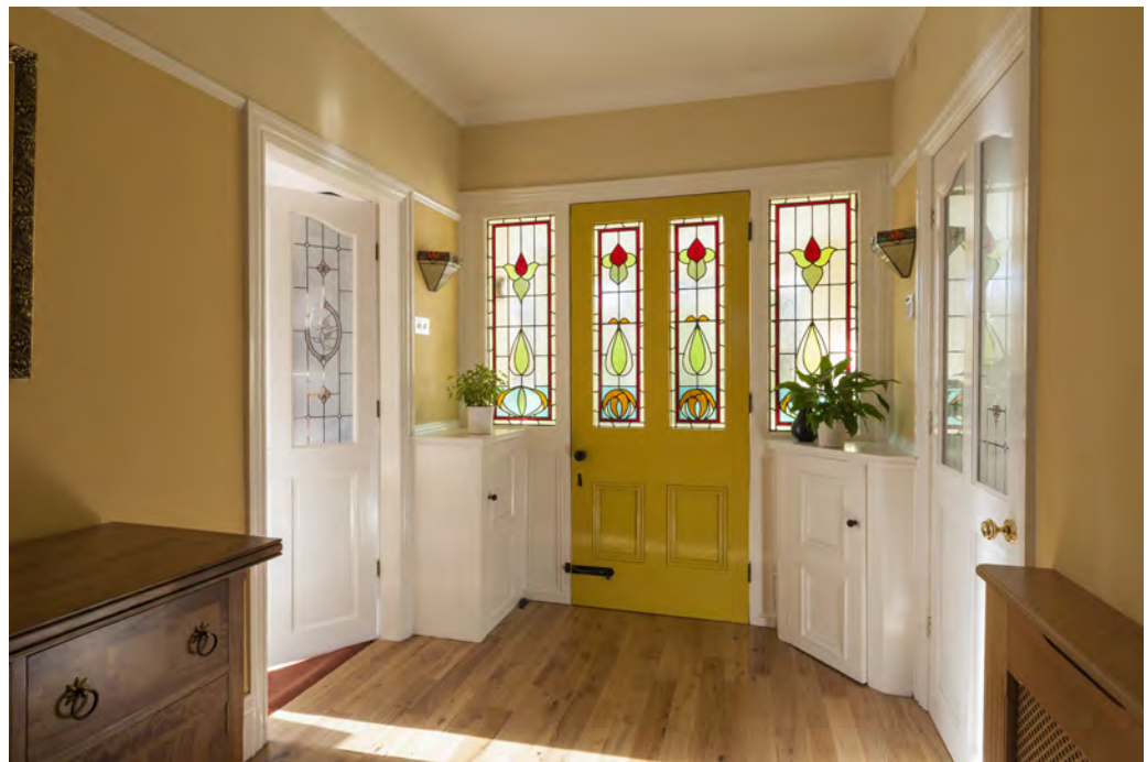
Figure 2-5-2: Stained glass in homes is not very common, but when it is installed, it is often only in showcase areas, such as a front door sidelight or a transom over a picture window. The probability of hazard is reduced, so the IRC allows the design freedom.
