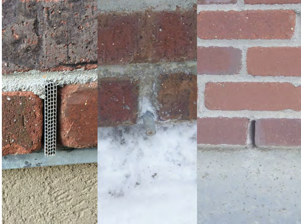
Figure 2-3-7: Weepholes for anchored veneers come in a variety of styles, sometimes corrugated plastic, a tube, a wick, or even simply not grouting a head joint. These can open onto a deck or below, just not into the back of a ledger or beam.
