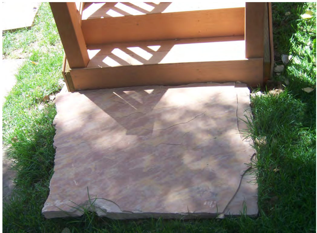
Figure 8-1-7: Flagstone is an effective landing material to balance the minimum safety necessary for stairs with an attractive transition from decking materials to natural landscape materials. There is no requirement for a concrete landing.
