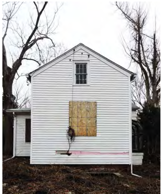
Hole in wall at West elevation Photo No. 6
