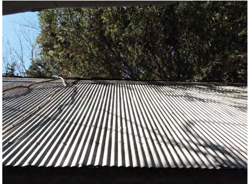
Building No. 3 - Existing corrugated metal roof Photo No. 29
