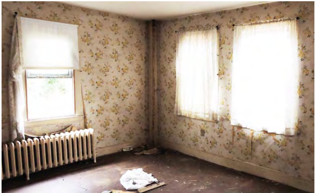
Front Parlor. Evidence of water infiltration below windows. Photo No. 7
