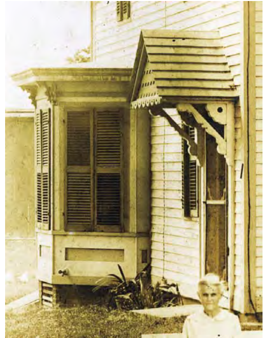
Figured brackets and fancy cut shingles at entry Photo No. 3
