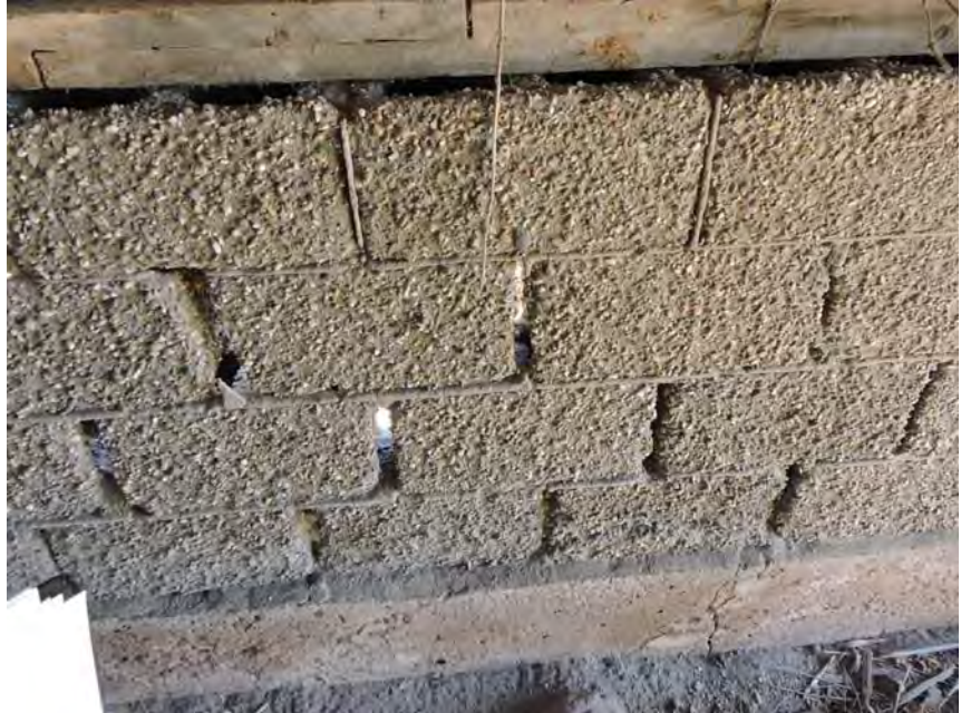
Building No. 2 - Erosion at concrete block foundation walls. Photo No. 27
