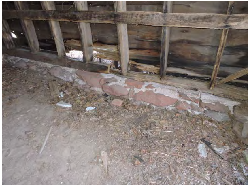
Building No. 5 - Note condition of timber sills. Photo No. 35
