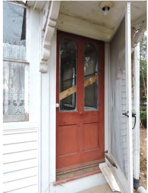
Door 'B' at South Entry storm door head lower than door head Photo No. 11B
