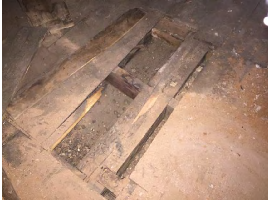
Main Attic - no insulation below floorboards of main attic. Photo No. 16
