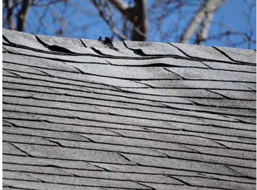
'Divot' at ridge where original chimney was roofed over Photo No. 18
