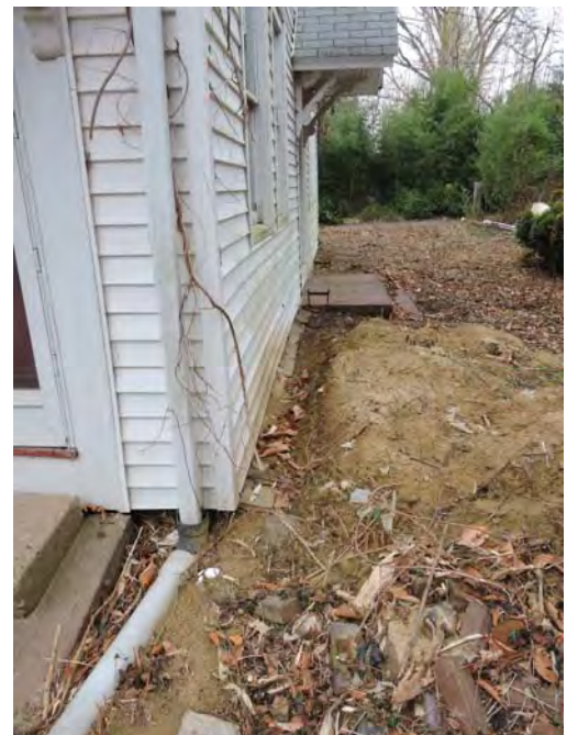
Grade is too close to sill at the East elevation (even without the pile of sand) Photo No. 4
