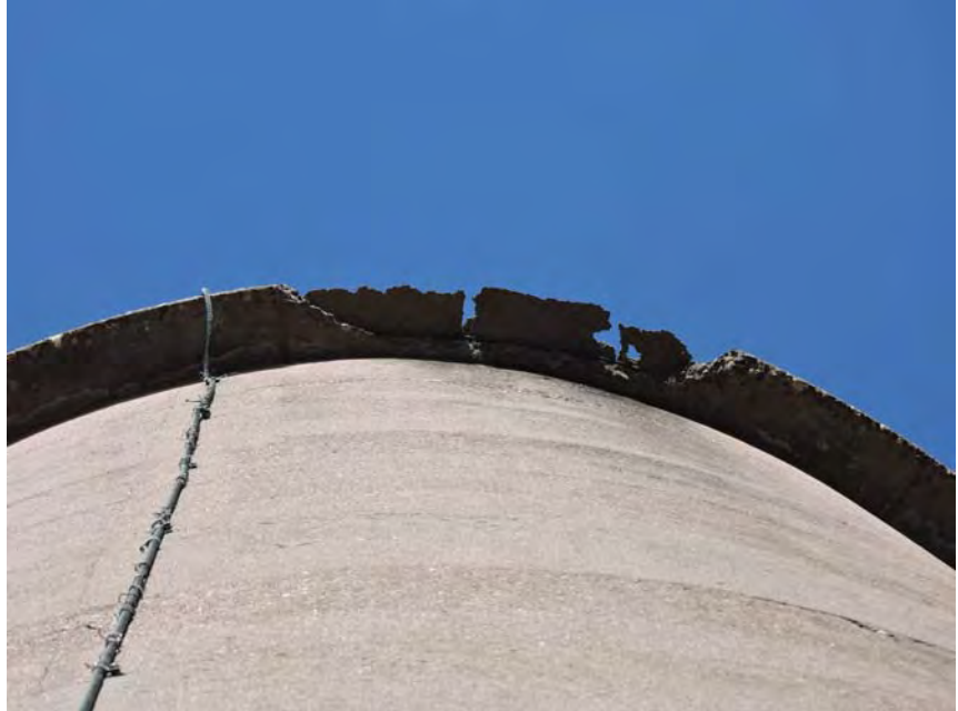
Silo - spalling at the roof overhang. Photo No. 39
