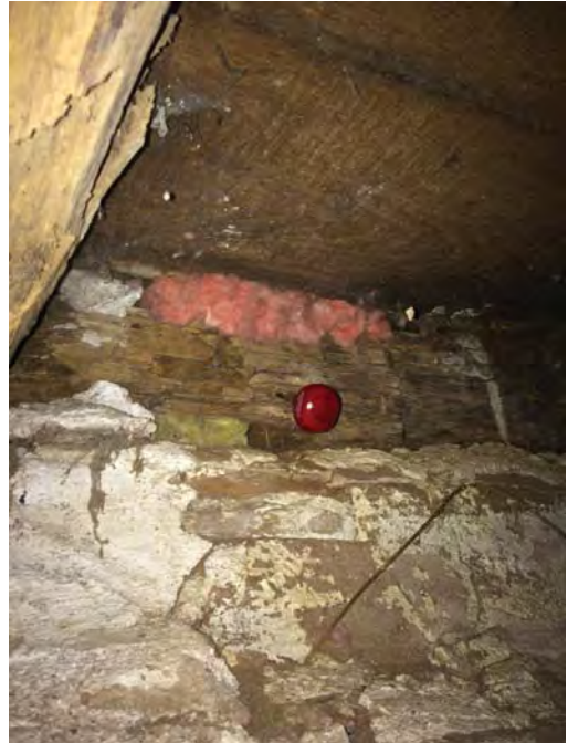
Awl pushed into deteriorated stretch of timber sill. Photo No. 5
