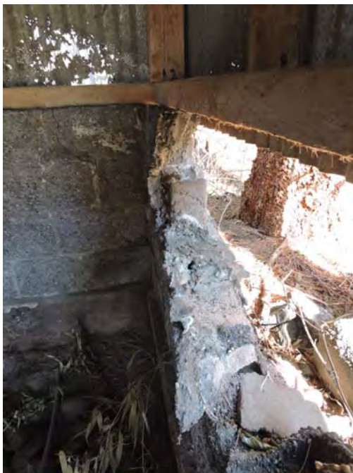
Building No. 2 at NE corner. Noted pitted metal siding, damaged foundation. Photo No. 25
