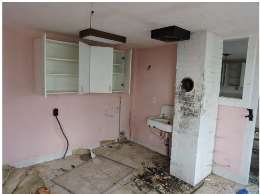
Metal pipe chimney connection; wood stove previously removed or stolen. Photo No. 19
