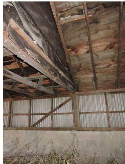
Building No. 2 - interior 'gable end' suggesting the roof structure may have been salvaged from another building. Photo No. 26
