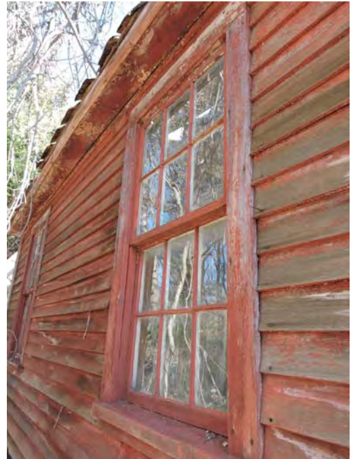
Building No. 1 - Double hung window on West elevation Photo No. 22
