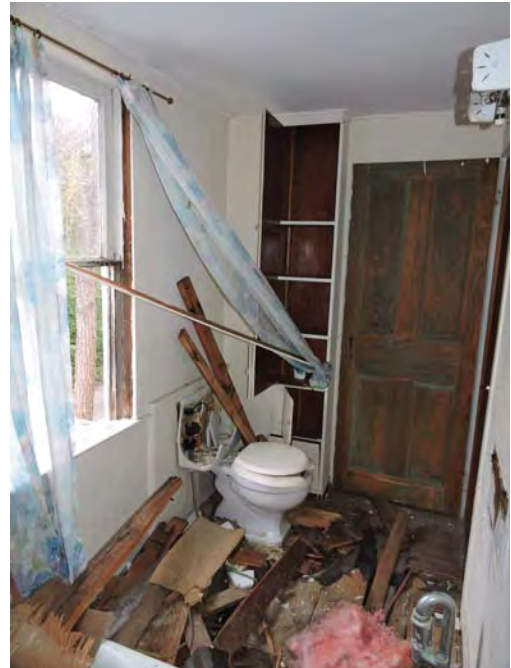
Plumbing in upstairs bathroom was raided by vandals. Photo No. 20
