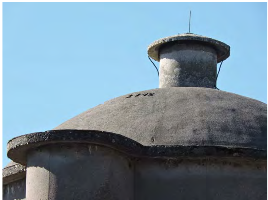
Silo roof dome. Note crack to the right of the date, as well as existing lightning protection system. Photo No. 38
