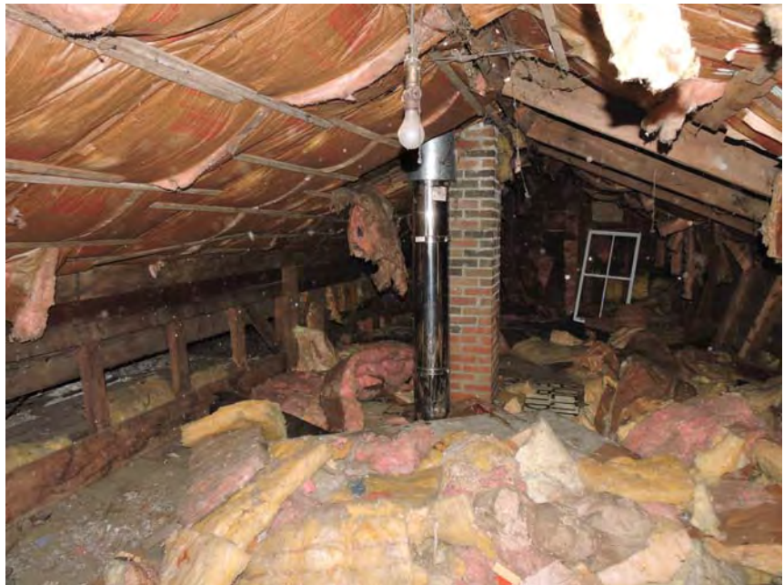
West Ell attic - batt insulation in disarray Photo No. 15
